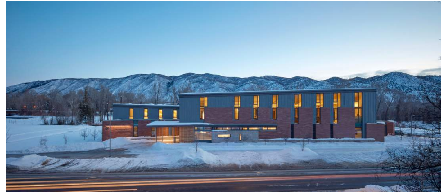
(Above) Rocky Mountain Institute Innovation Center utilized Factor 10 Engineering to further each sustainable strategy. The enhanced exterior envelope had a 4 year payback when considering it helped eliminate traditional mechanical systems and improved indoor environment quality resulting in increased productivity and engagement.
