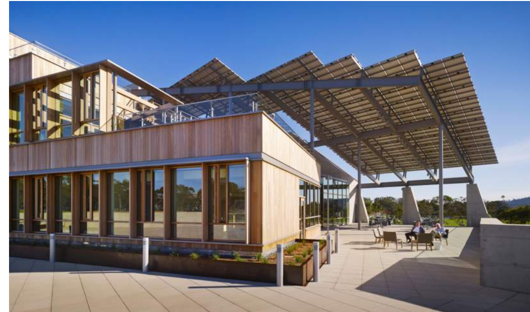
(Left) The J. Craig Venter Institute has two photovoltaic arrays comprising 26,124 SF of surface area that are predicted to exceed the building demand, pushing excess power generated back into the grid. These arrays are utilized as shading devices in most of the exterior spaces.
