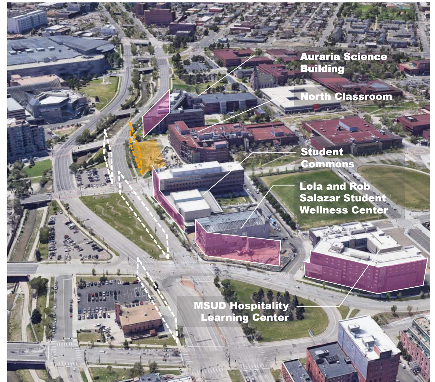
Aerial Image - Speer Boulevard Facades
