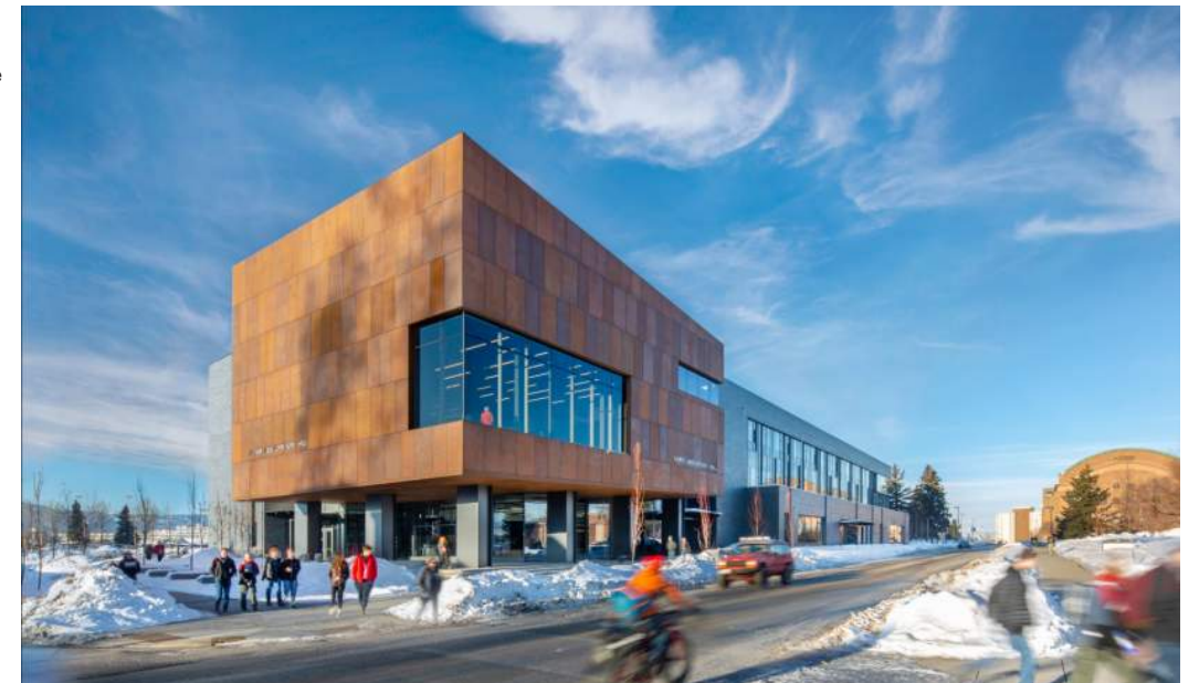
(Right) Montana State University, Norm Asbjornson Hall uses transpired walls to preheat outside air. Air passing through the transpired wall is preheated to 60 degrees in the middle of Montana's winter before entering the building. This effort is on track to save MSU millions of dollars in operating costs over the coming years.
