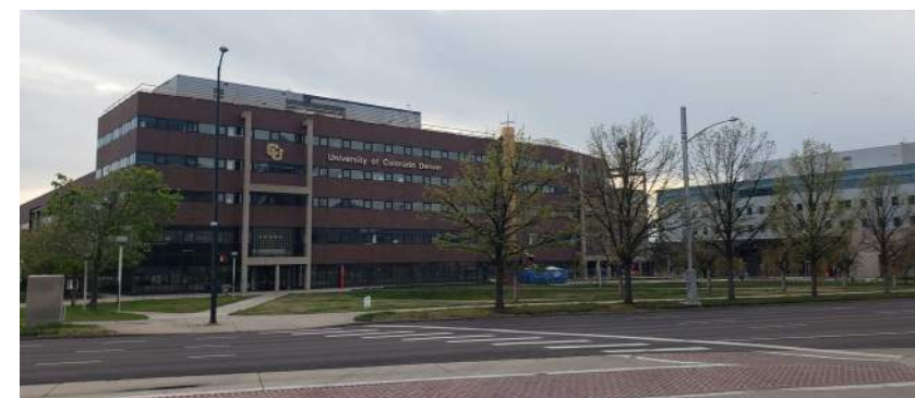
Site from Speer Boulevard and Lawrence Street
